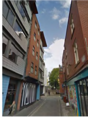
5 – Carpenters Lane – 5.5m
